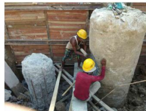
Pile Head checking
